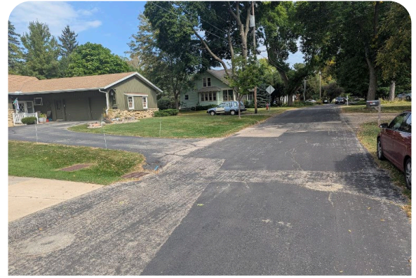
Pontiac Trail (looking north) Cars parked in the terrace and undefined drainage flow paths have worsened maintenance, flooding, and safety issues that this project aims to address.
