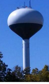
Madison water towers are usually painted with a one or two-tone color scheme. Two-tone schemes have been applied on some towers to help mask any mildew or rust that can be caused by condensation on the bottom of the tank.
