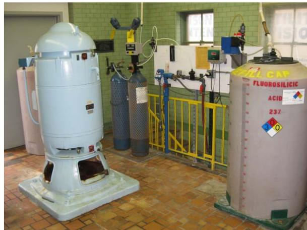
Figure 5-2: Well Pump for Well 7
