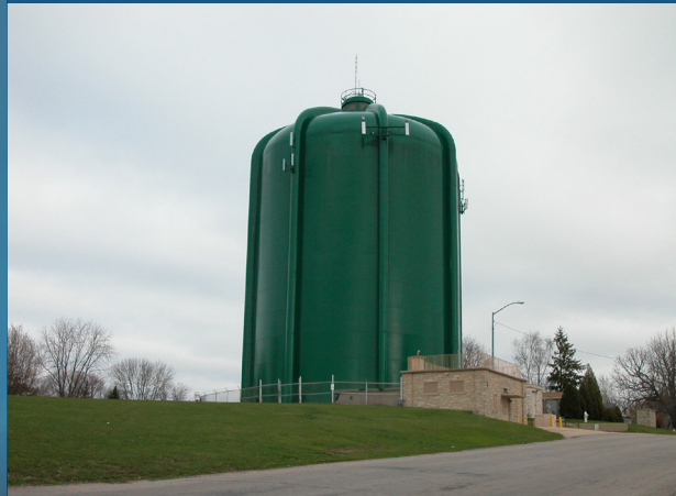
Unit Well #9 Pump Station Project Status: Completed | Investment: $100 thousand
