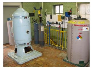
Figure 5-2: Well Pump for Well 7
