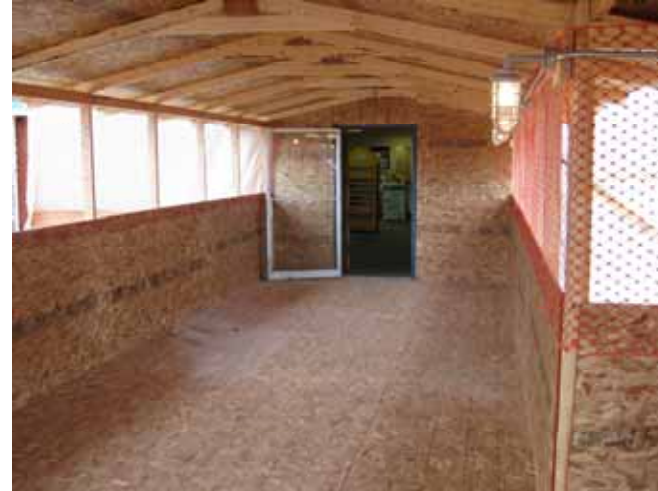
Picture above shows the walk path inside the new covered entrance.
