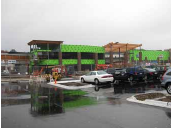
Picture above shows the new parking lot and Atrium Progress
