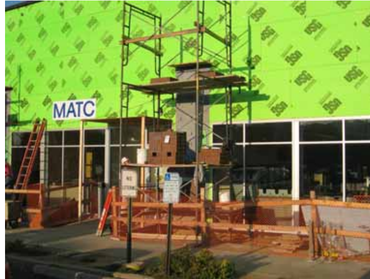
Picture above is new masonry columns under construction
