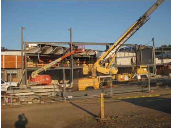
Picture above shows structural steel skeleton of the new Atrium!
