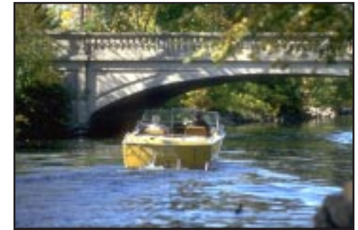
Rutledge Street Bridge looking northwest
