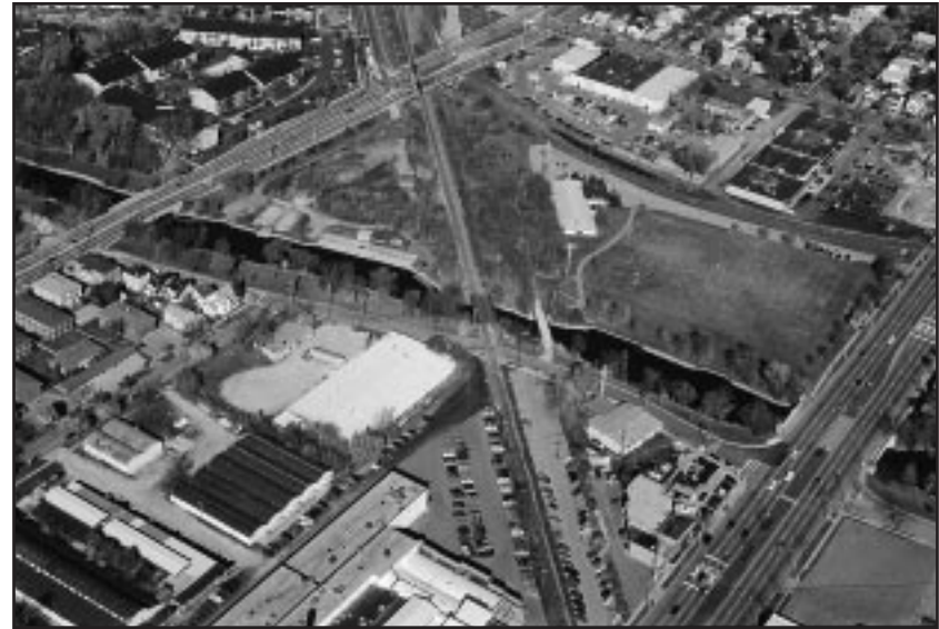
Looking north at the Burr Jones park site and the Yahara River
