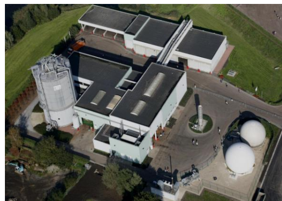
Wet anaerobic digestion facility (L) and dry anaerobic digestion facility (R) with pre- and posttreatment and energy production
