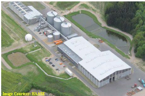
Wet anaerobic digestion facility (L) and dry anaerobic digestion facility (R) with pre- and posttreatment and energy production
