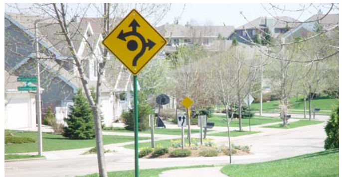
Permanent installation of a traffic circle at New Washburn way and Dandaneau Trail
