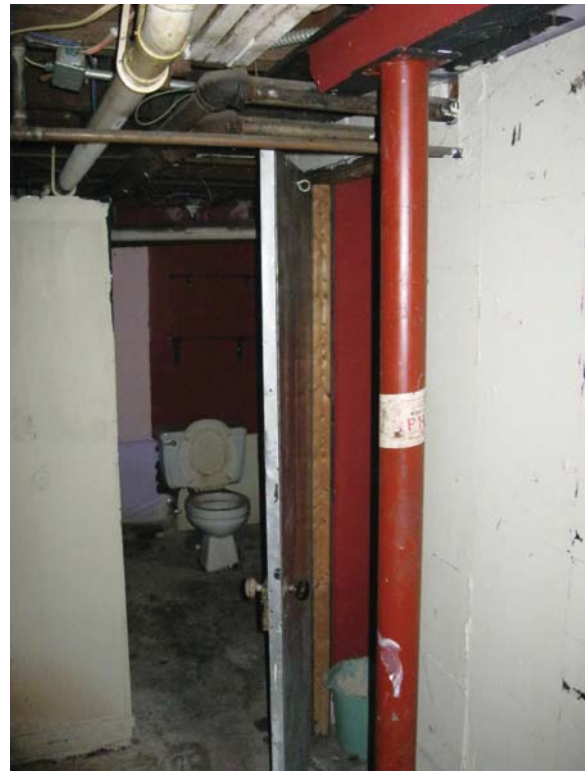
Photo 10 – 1 st floor shoring beam and post
