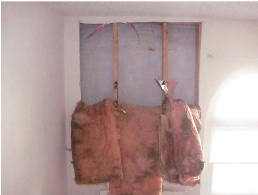
Figure 12. Staining and evidence of moisture penetration was observed on the batt insulation and plaster at an inspection opening created at the third floor during the site visit.
