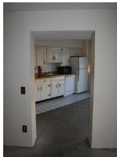
Second Floor: Structural bearing wall between living room and kitchen
