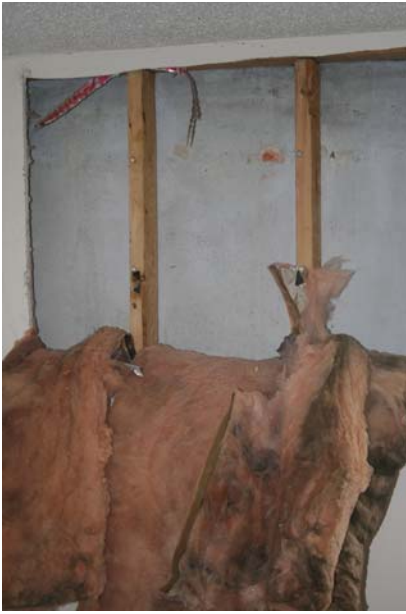
Third Floor: Section of exterior wall exposed showing back of brick and moisture within the insulation space
