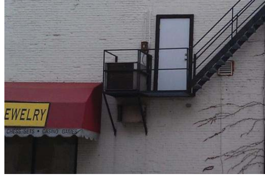
Apartment condensing unit
