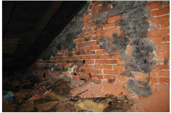
Attic: View toward wall between 127-129 state street and the castle and doyle building showing significant damage to existing brick
