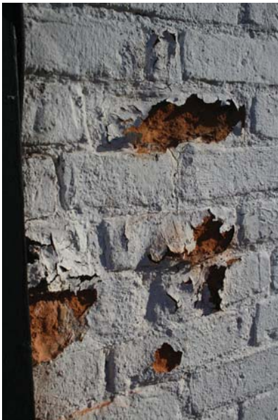
Exterior: View of damaged brick veneer
