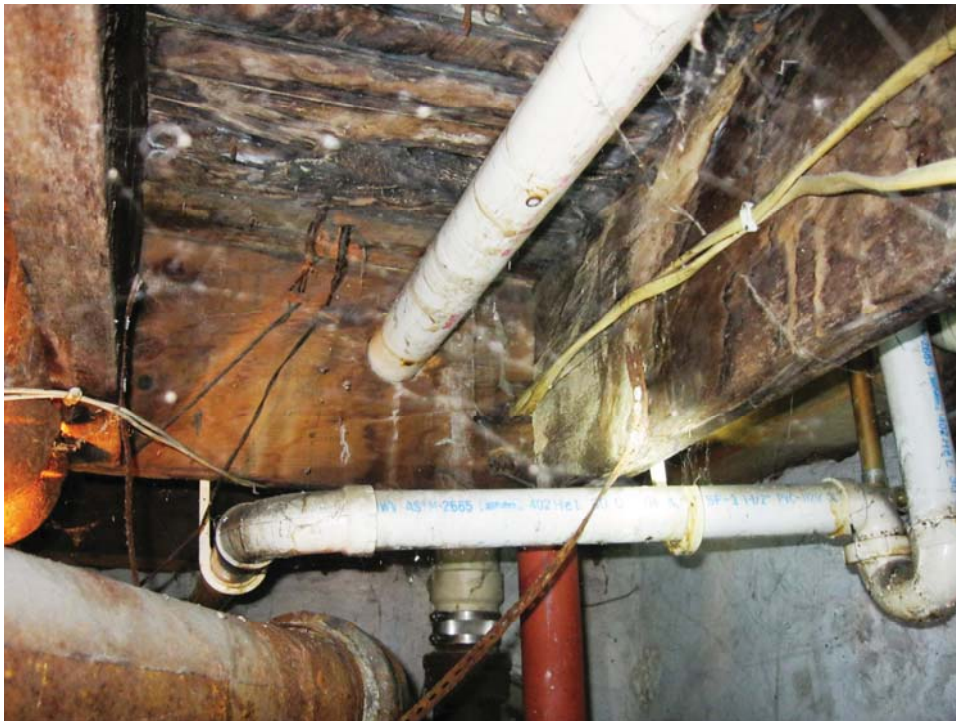
Photo 7 – 1 st floor framing with water damage
