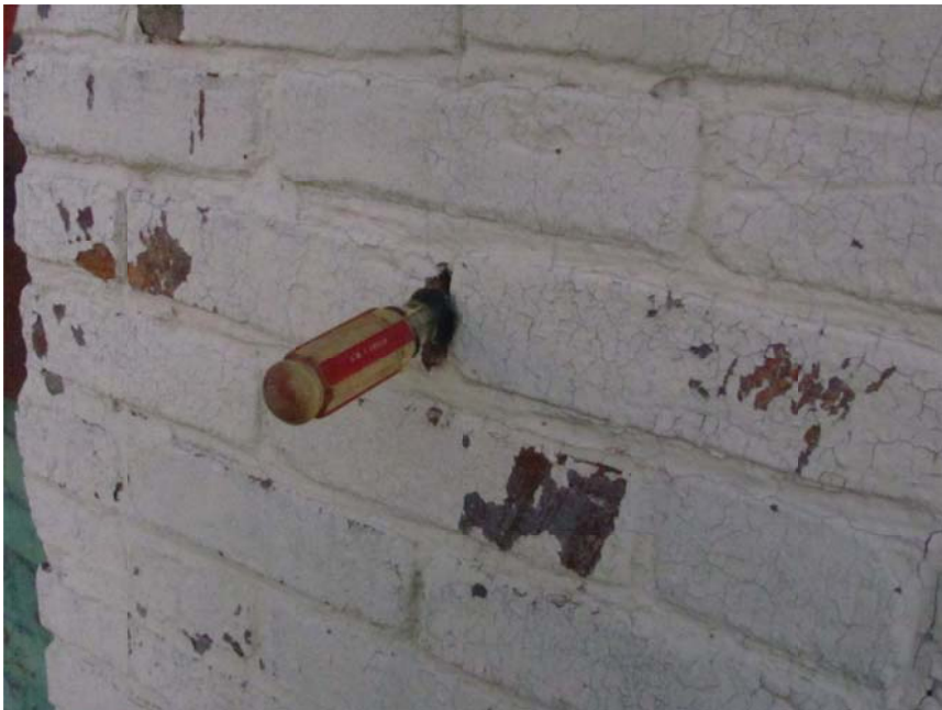
Figure 6. Mortar behind the coating layers has disintegrated, resulting in voids within the masonry construction.
