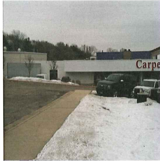
Adjacent East Building (Carpetland)
