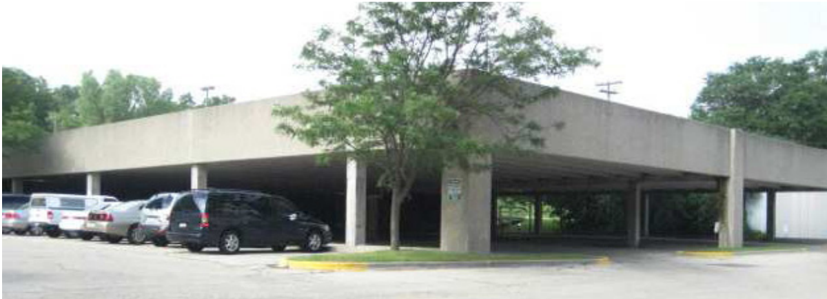
610 N. Whitney Way, "PSC Parking Ramp"
