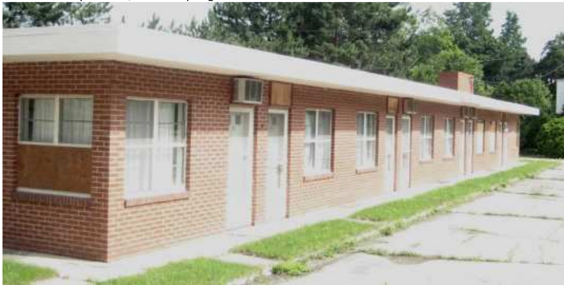
5119 University Avenue, "Quonset Hut"
